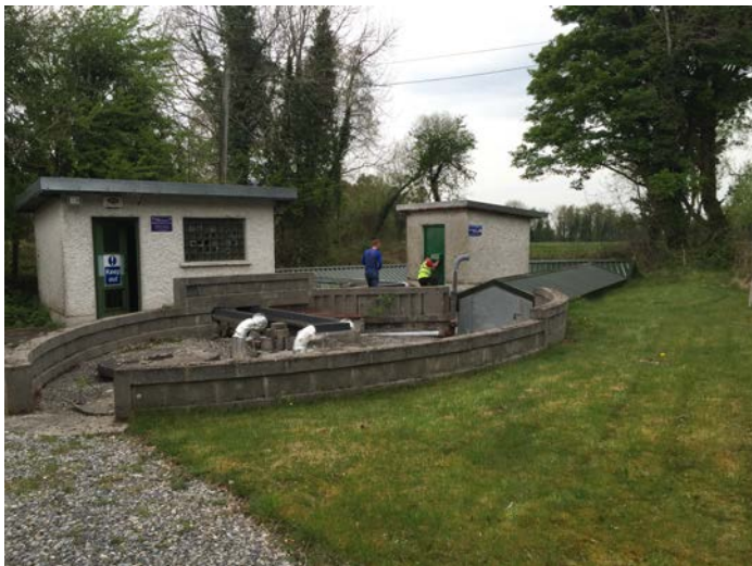
Photo 1 – Toberfin Springs – Killeigh, Killurin and Cloneygowan GWS Pump House on the left of the image; Meelaghans GWS Pump House on the right of the image
