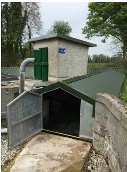
Photo 2 – Toberfin Springs – Killeigh, Killurin and Cloneygowan GWS long metal shed covering the springs
