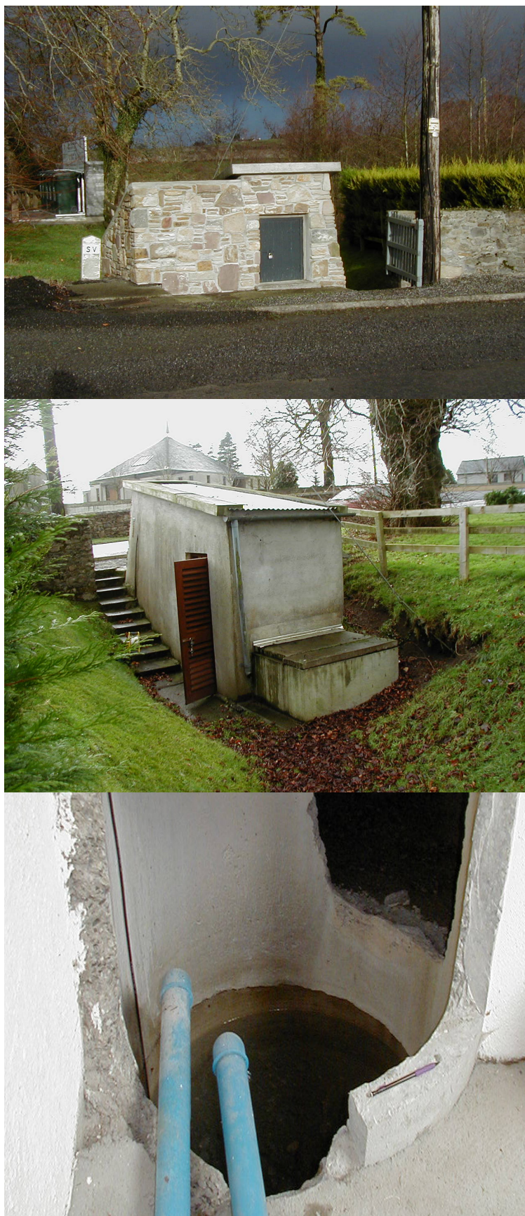
Figure 1 Views of Dunkerrin Village Well Pumphouse and Chamber
