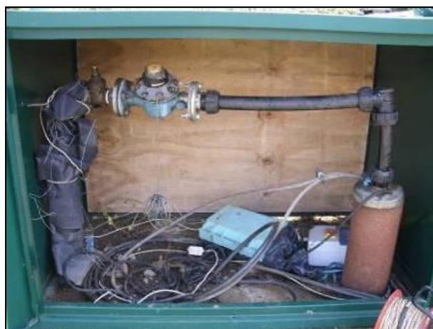
Photo 2: Well Head Construction (BH-1)
